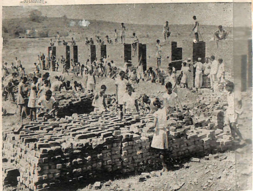
Members of the Bhopal Armed Constabulary lending their hand in the construction of a Police Children's School.
